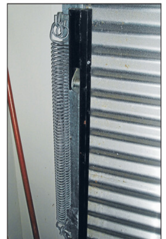
Tension: Garage door springs should be serviced every year or two, a door fitter advises.
